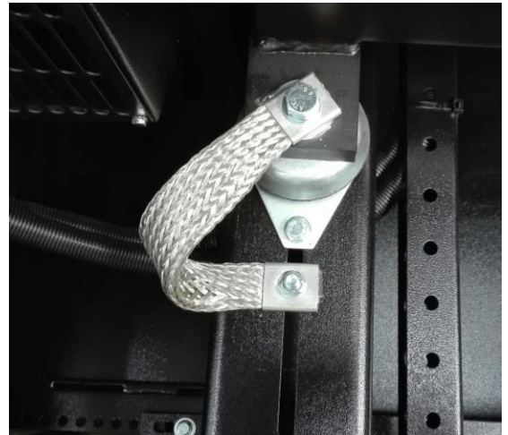
Fig. 4.1: Ground connection of internal components
