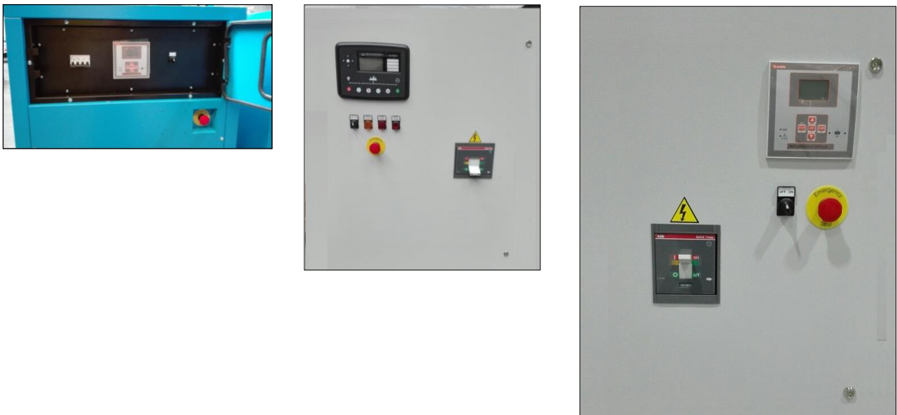
Fig. 3.4: Some examples of automatic control panels
