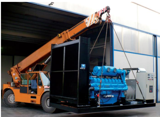
Fig. 7.2: Lifting the generating sets by means of lifting hooks.
